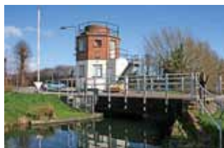
Bond Mill Bridge today
