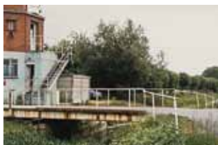
Bond Mill Bridge, 1986
