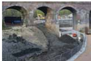
Capel's Mill under restoration
